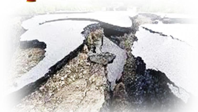
An aerial photograph showing a severely damaged asphalt road. The road is split into several large, jagged sections that have shifted and broken apart, with deep cracks and exposed aggregate. The surrounding area appears to be a mix of dirt and asphalt, suggesting a recent earthquake or similar geological event.
